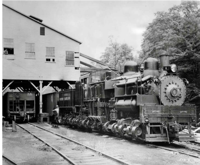
Western Maryland three-truck Shay No. 6 works a coal plant on the Chaffee (W.Va.) Branch not long after delivery in 1945. The 324,000-pound giant was the last of nearly 2,800 Shays built by Lima Locomotive Works. Today it works on the Cass Scenic Railroad. Western Maryland photo
