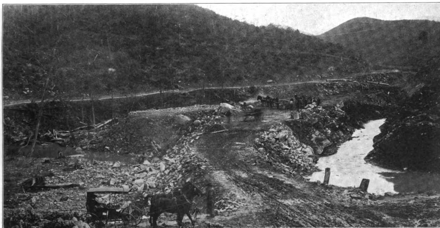
Laurel Branch, near Pocahontas; Change of Creek Bed Saves Two Bridges.
